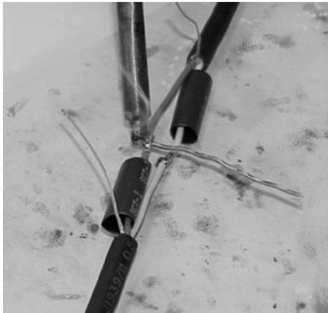
Solder Wires Together
